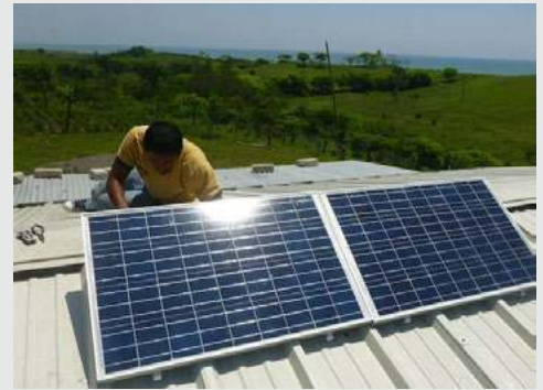
A worker installs a rooftop solar panel. Image credit: Ilumexico
